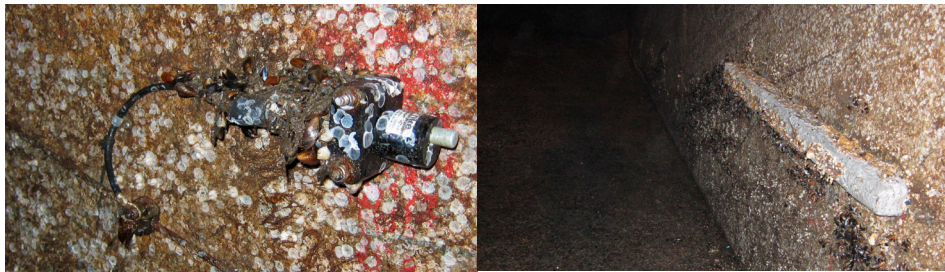
Figure 5: The potential logger mounted on the concrete wall is shown to the left and an sacrificial anode mounted on the concrete wall is shown to the right.
